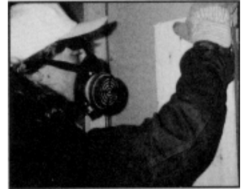
Wear protective clothing and a respirator when removing walls that may contain lead.
